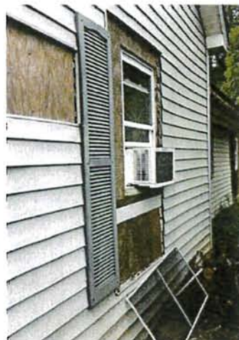
Plywood covering old window openings (re-sized)
