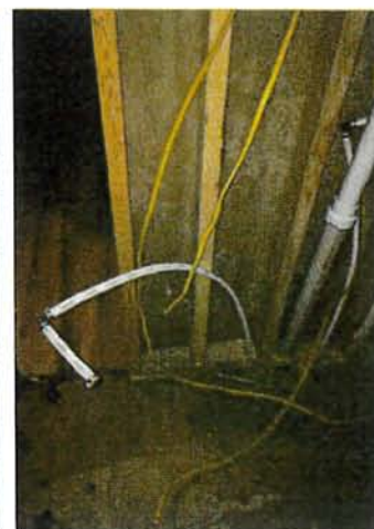
Exposed water lines
