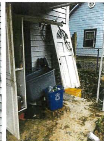
exterior storage, building materials
