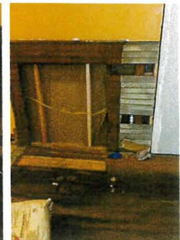
open wall from former chimney
