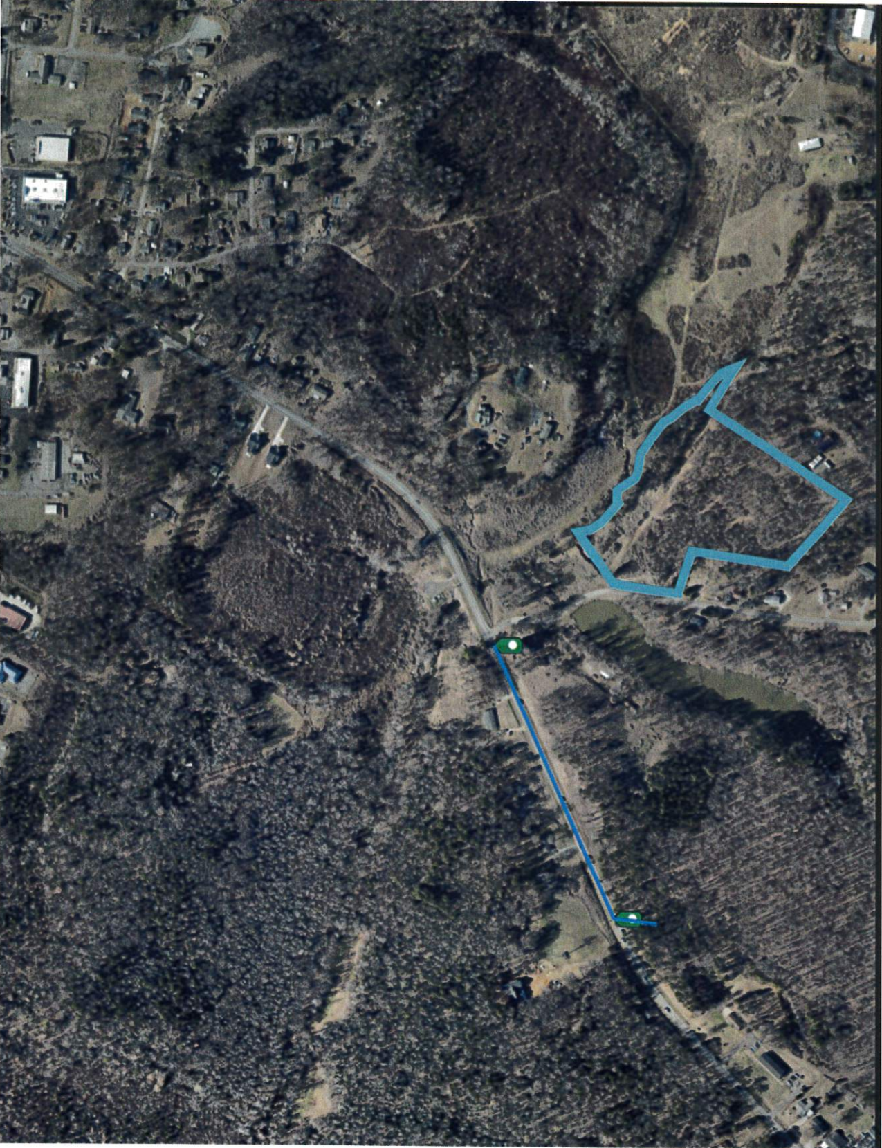
Aerial Below shows approximately 1,000 ft beyond Evans Lake Road near 638 Dallas Stanley HWY.
